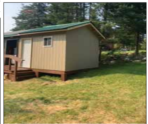
New Laundry Building
